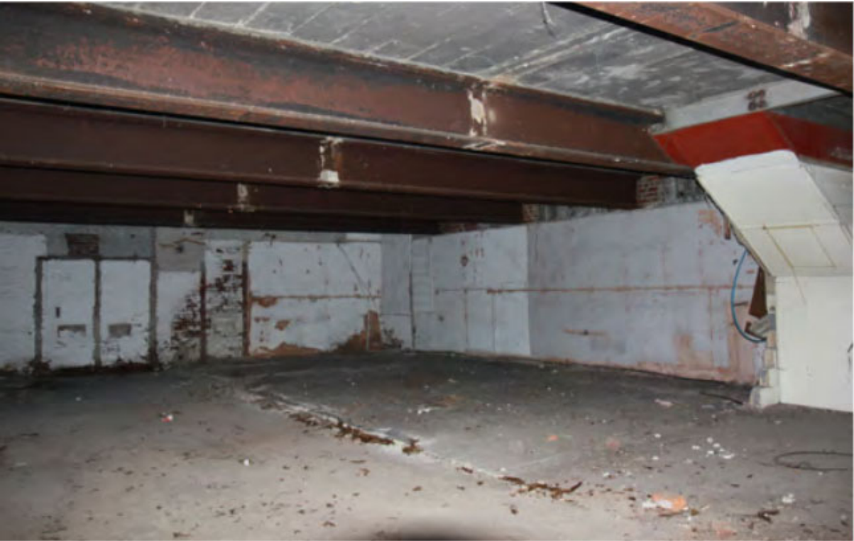
Boiler House Ground Floor interior 2016
