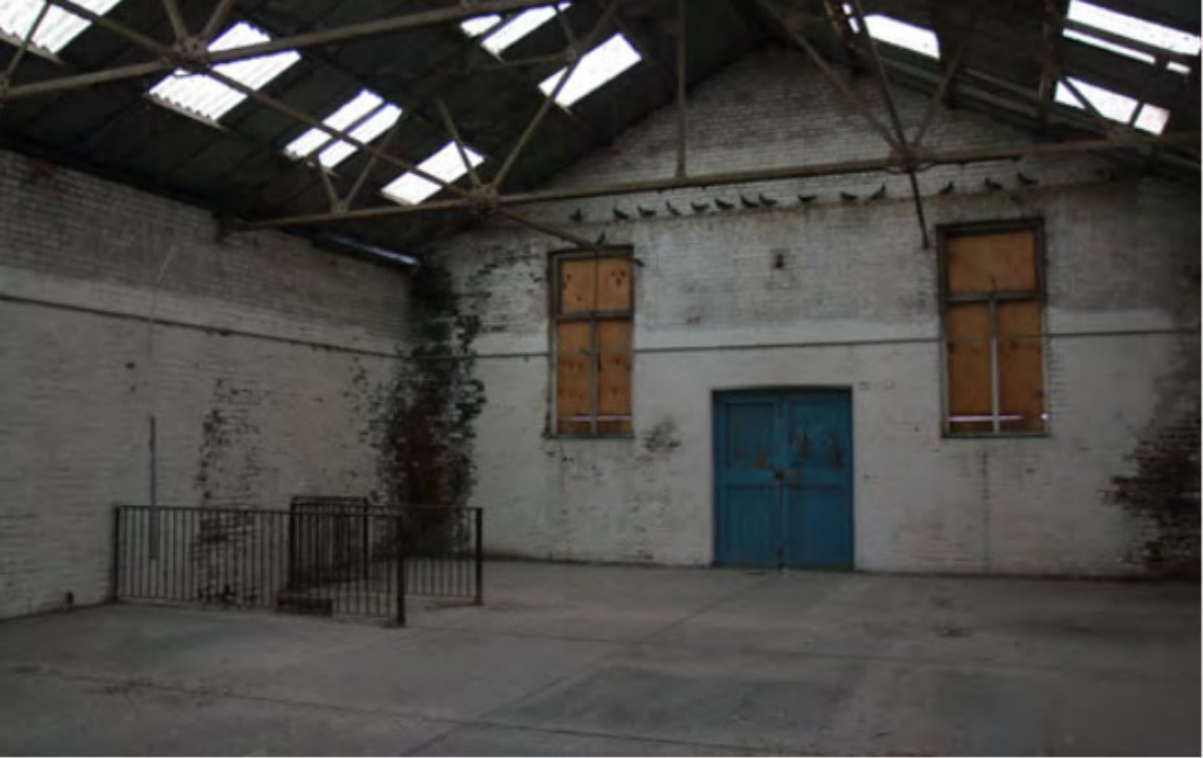
Boiler House Upper Level interior 2016
