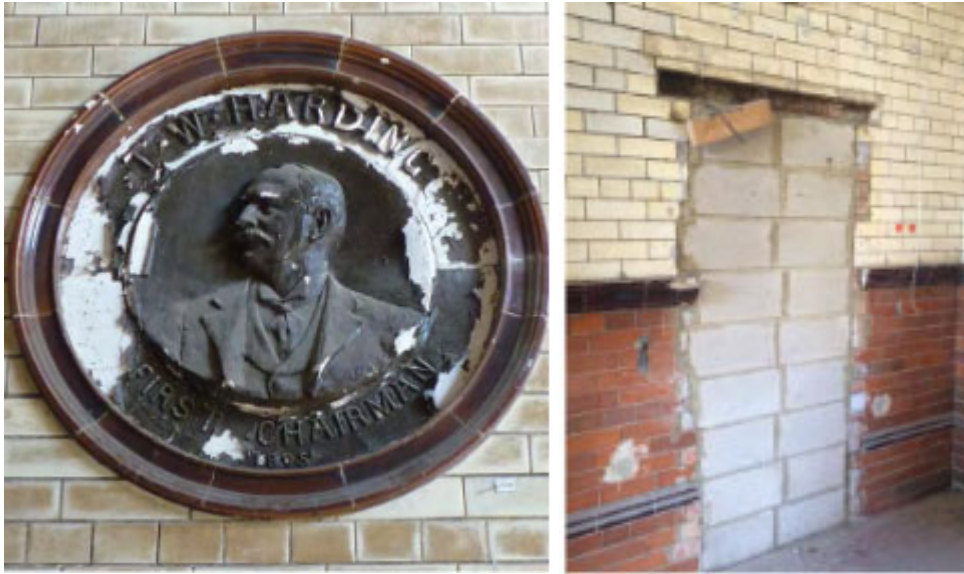
Medallion detail, and Burmantofts glazed brickwork - 2016
